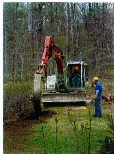
Trenching to break grafted roots
